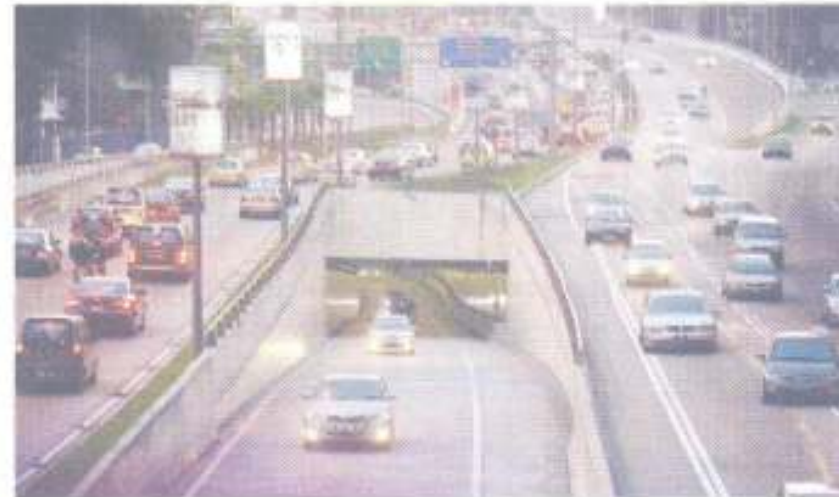
Smooth flowing: A file picture of the SMART tunnel.
