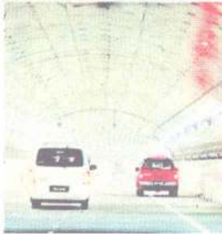
The SMART tunnel is a man-made wonder!
